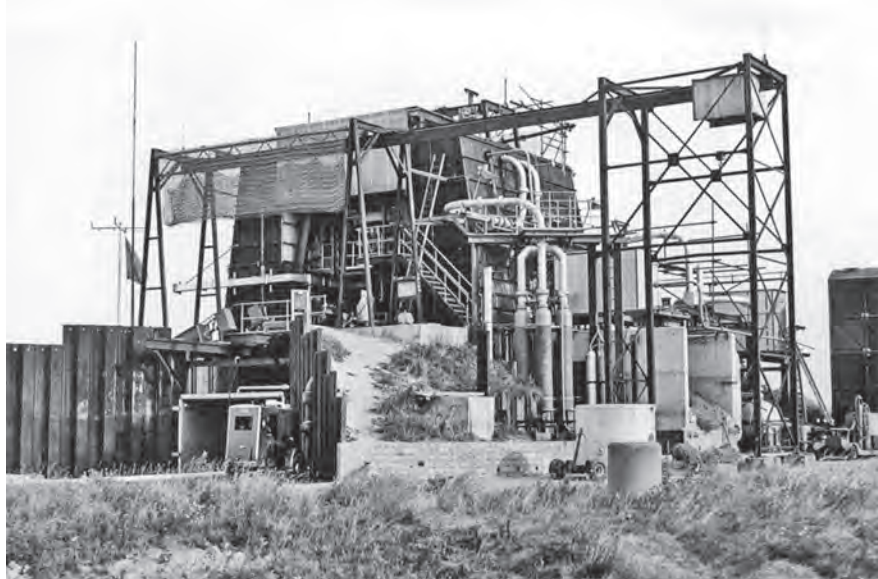
P 2 Site; P1 is seen to the rear
